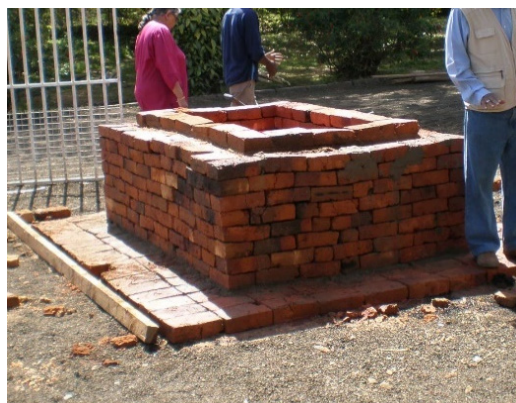
ZECC: A simple brick and sand structure constructed using a double brick wall with the space between the two walls filled with moist sand.
